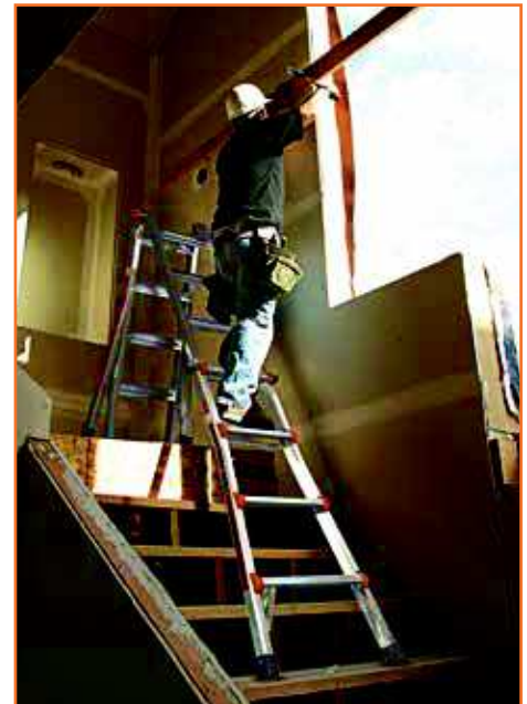
Safe, easy stair access.
